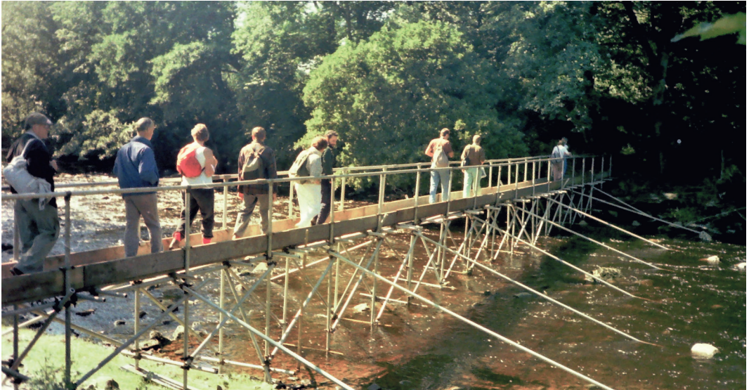
Figure 44. The temporary bridge erected over the river Irthing at Willowford
