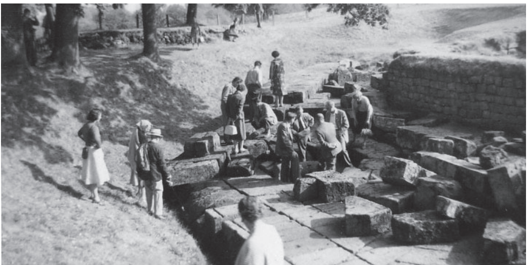
Figure 36. Chesters bridge abutment
