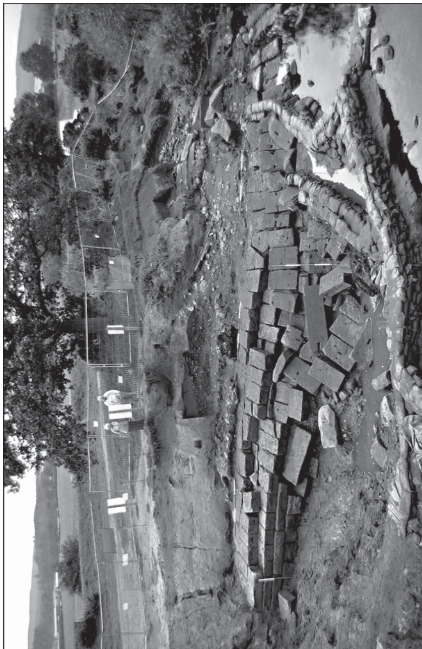
Figure 25. The S road ramp of the Roman bridge at Corbridge, under excavation in 2004
