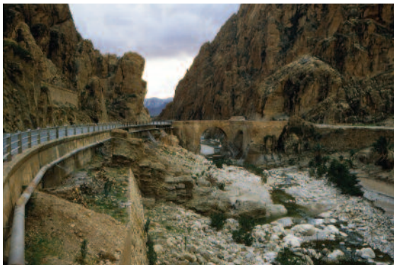
108. Roman bridge in the al-Kantara pass, connecting the Aures High Plains near Lambaesis with the pre-desert zone (Algeria)
