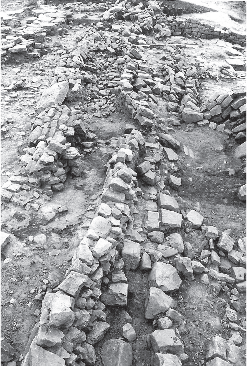
Figure 4.33: North rampart revetment walls at Housesteads dating to the mid-late 4th century. Source: Alan Rushworth.
