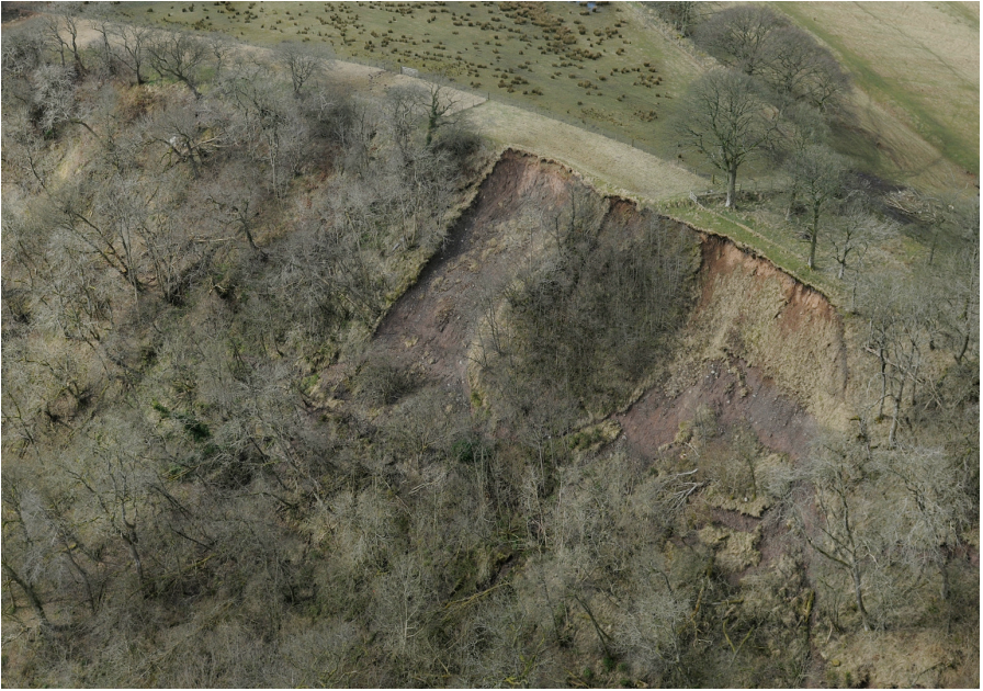
Figure 4.45: Aerial photograph of erosion scars beneath the cemetery at Birdoswald. The pale grassed area on the edge of the cliff was totally excavated. Source: Historic England.
