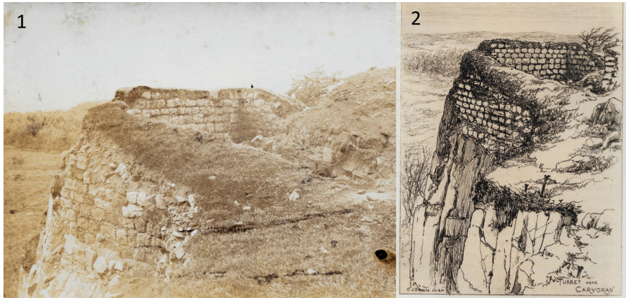
Figure 4.42: A photograph dating to the 1880s of turret 45b (1) compared to the illustration of the same turret by C.J. Spence. Source: TWAM (photograph), Society of Antiquaries of Newcastle upon Tyne (illustration).
