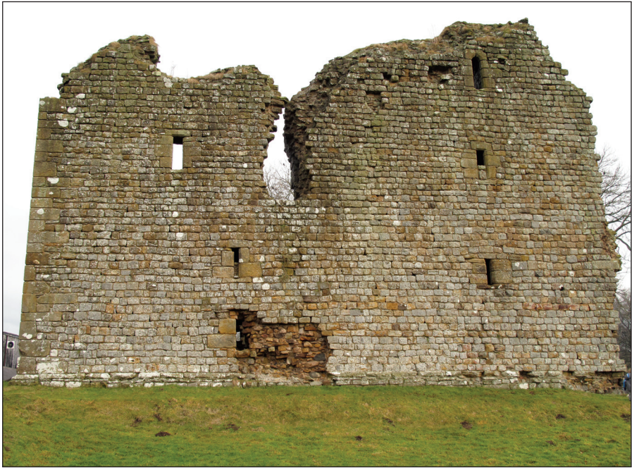
Figure 3.19: Thirlwall Castle, west of the fort at Carvoran and immediately north of the Wall, is built almost entirely of facing stones quarried from the Wall, and possibly rubble from the core of the curtain as well. Source: Rob Collins.
