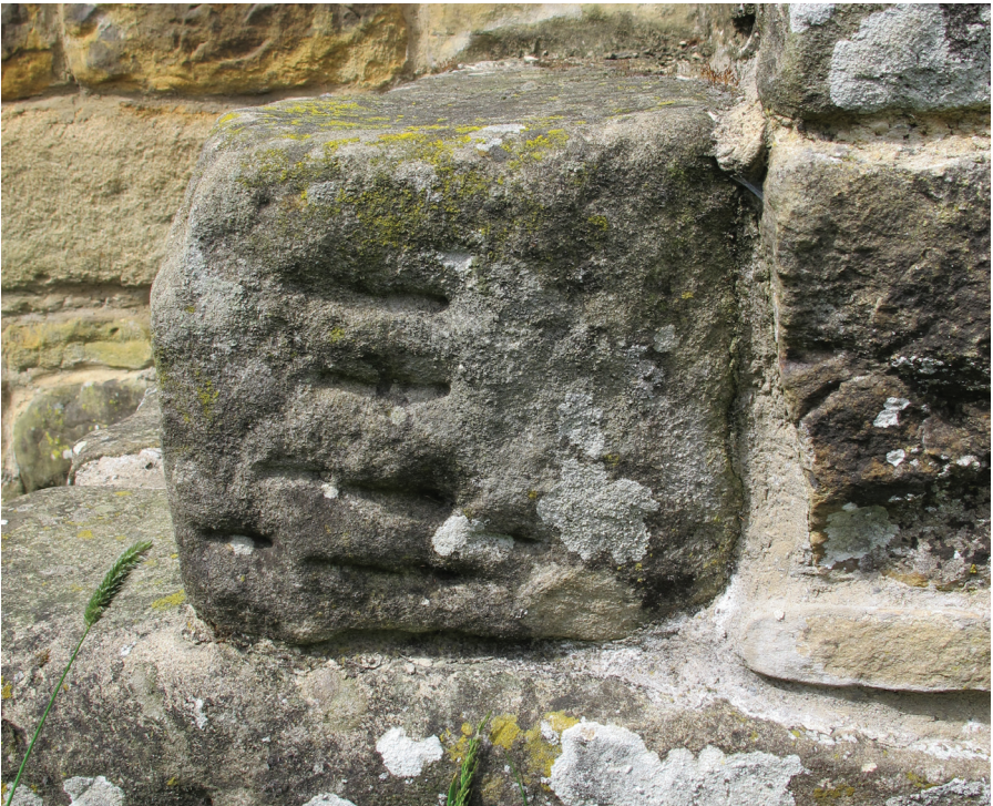
Figure 4.29: A shaped stone that is likely to be a voussoir and was found built into an external staircase of a barn at West Uppertown Farm. This stone is one of at least 13. Source: Lindsay Allason-Jones.
