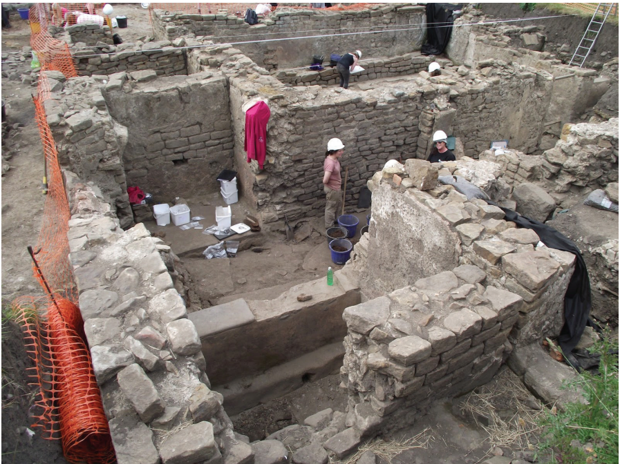
Figure 3.14: The extramural baths at Binchester were preserved due to the raising of the exterior ground level of Dere Street relative to the interior spaces, which were filled with rubbish in the 4th century, allowing the walls to survive to a height in excess of 2m. Source: ASDU.
