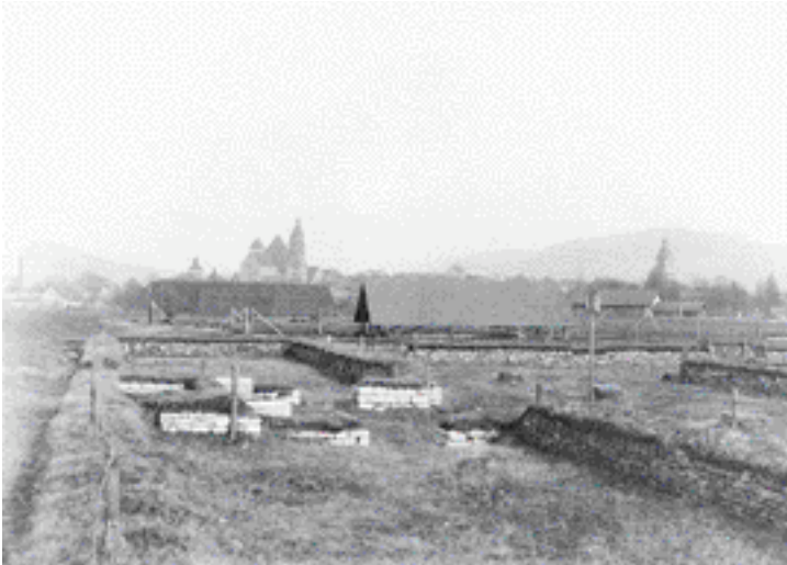
Fig. 1 Weißenburg i. Bay., Germany. Consolidation of the walls of the principia of the fort and protecting roofs around 1900, in the background the station (Photo: Archive of the Reich-Limeskommission, Römisch-Germanische Kommission of the Deutsche Archaeological Institute)
