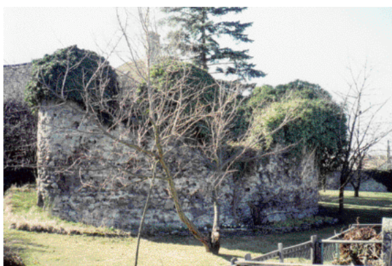
Fig. 3 The north-eastern fan-shaped tower, fort Zeiselmauer in 1986 (Photo: S. Jilek)
