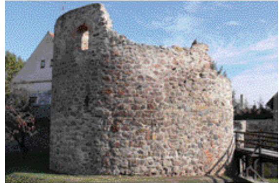
Fig. 7 The late Roman tower at the fortress Mautern in Austria, which still stand 2 storeys high (Photo: Boundary Productions)
