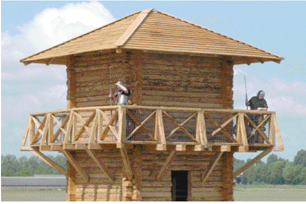
Fig 1 Reconstructed watch-tower near Utrecht (NL)
