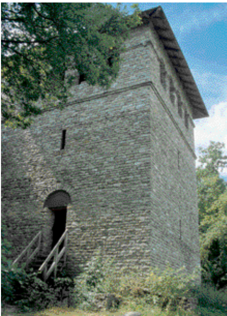
Fig. 7 The reconstructed watch-tower of Erkertshofen on the Upper-German Raetian Limes (Photo: A. Thiel)
