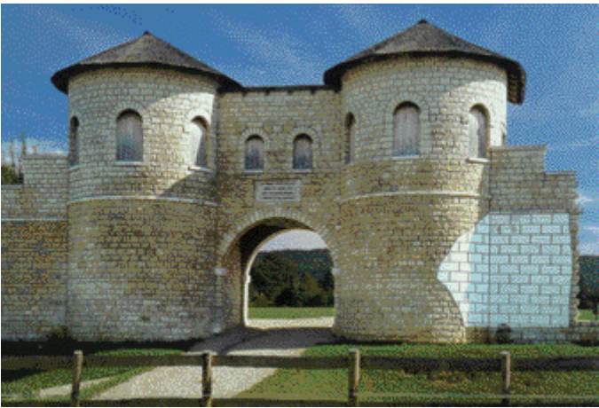
Fig. 3 The reconstructed gate in Weissenburg, Bavaria (Photo: BLfD)
